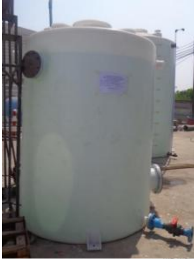
Flocculation Tank - 4m 3
